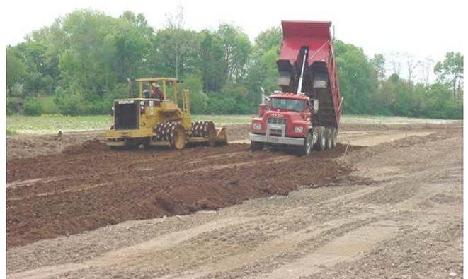
**Milestone raises the subgrade by placing and compacting fill**
